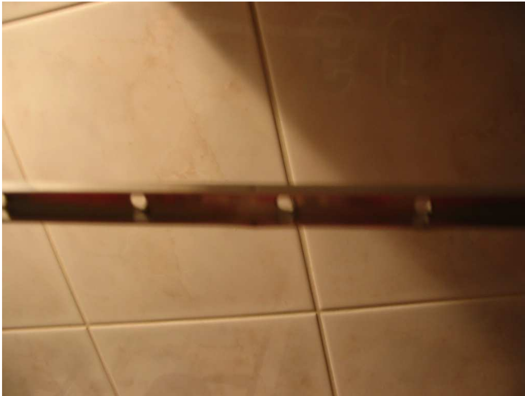
Image 14: Drilled holes in aluminum U-frame
